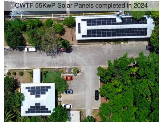
CWTF 55KwP Solar Panels completed in 2024
